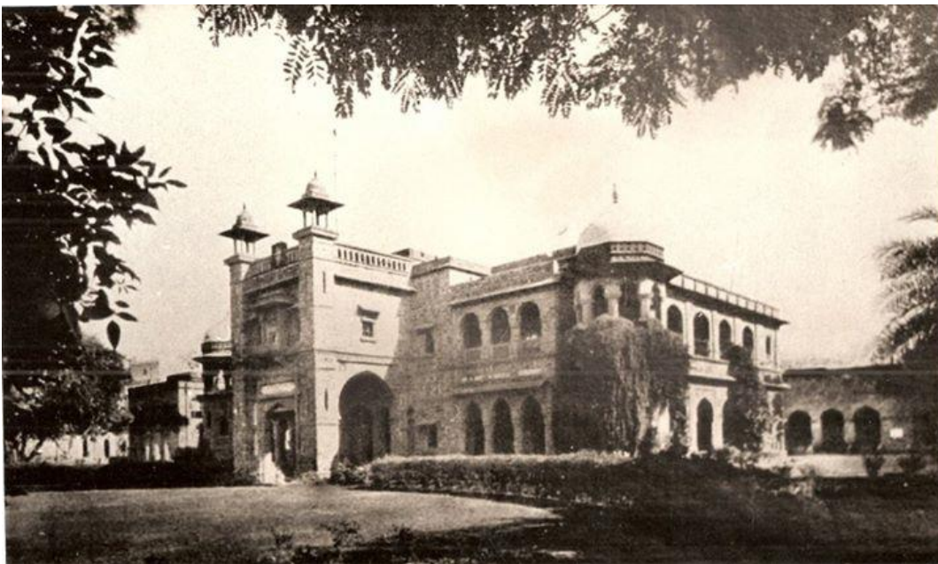
St. Stephen's College building at Kashmere Gate (Circa 1922).
